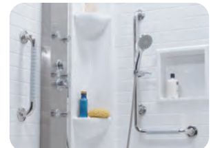
Built-in Grab Bars for Safety
